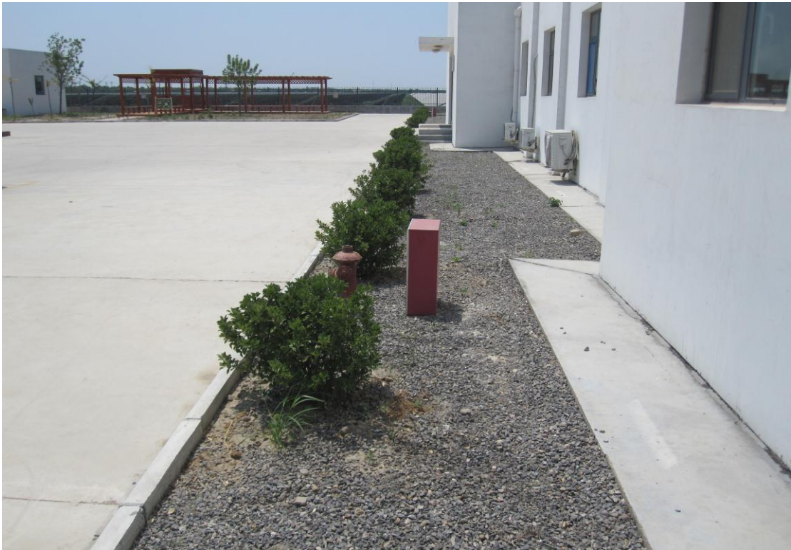
撒铺碎石防护
