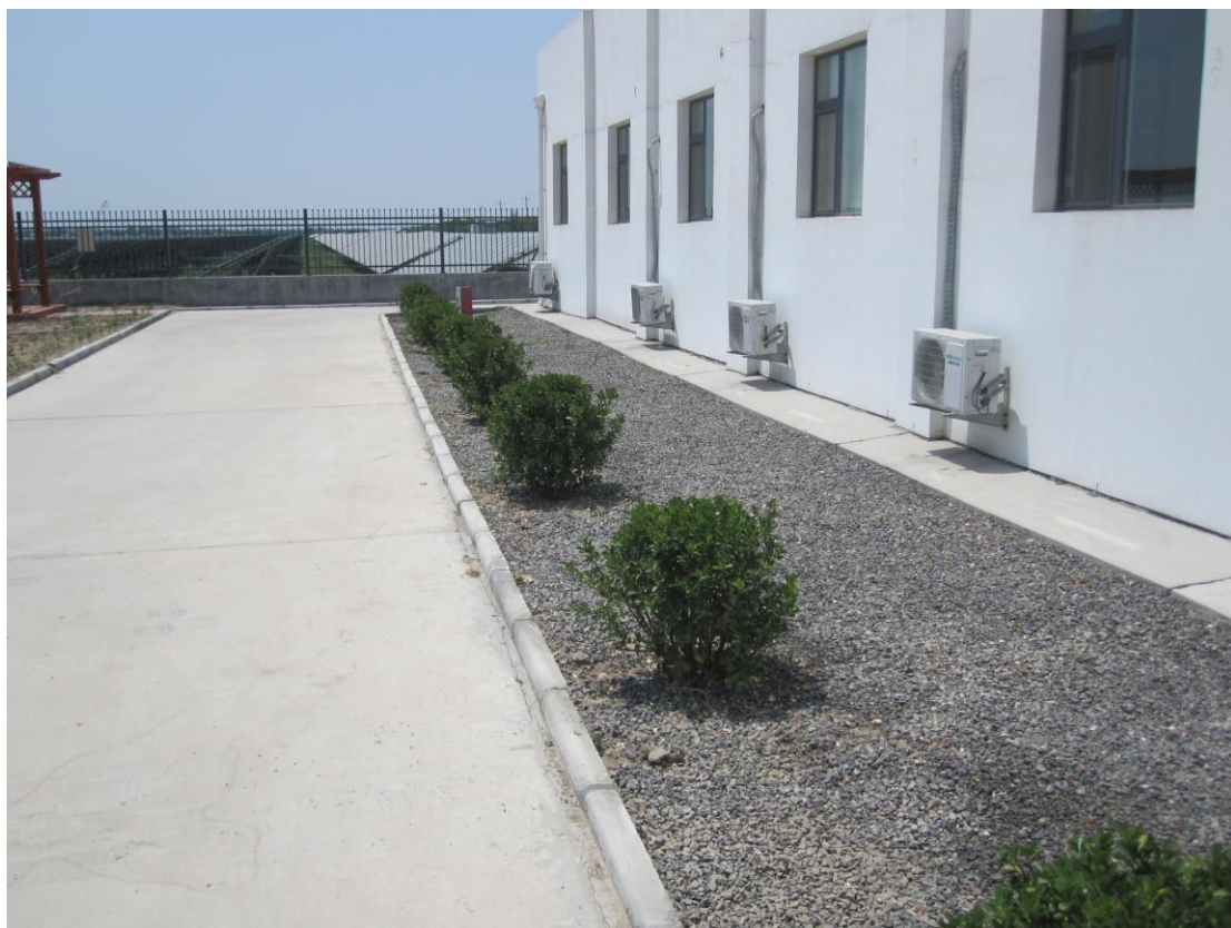
撒铺碎石防护
